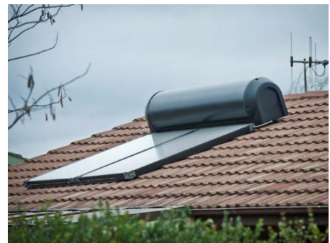
Thermosiphon solar water heater
